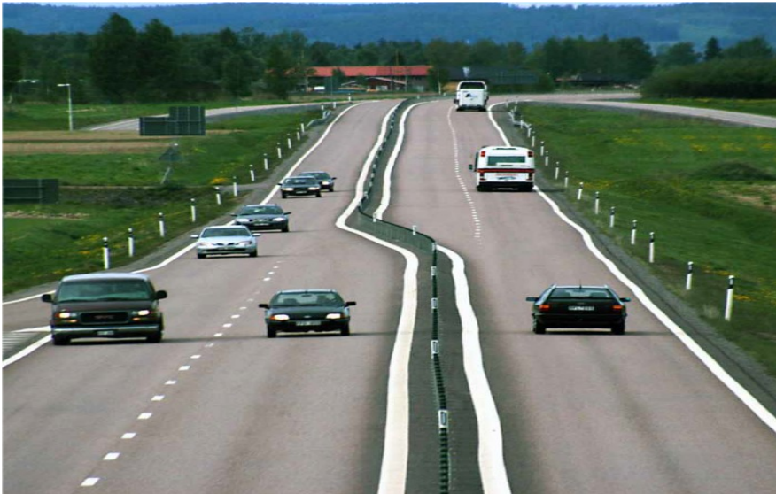
TRAFIKVERKET SWEDISH TRANSPORT
