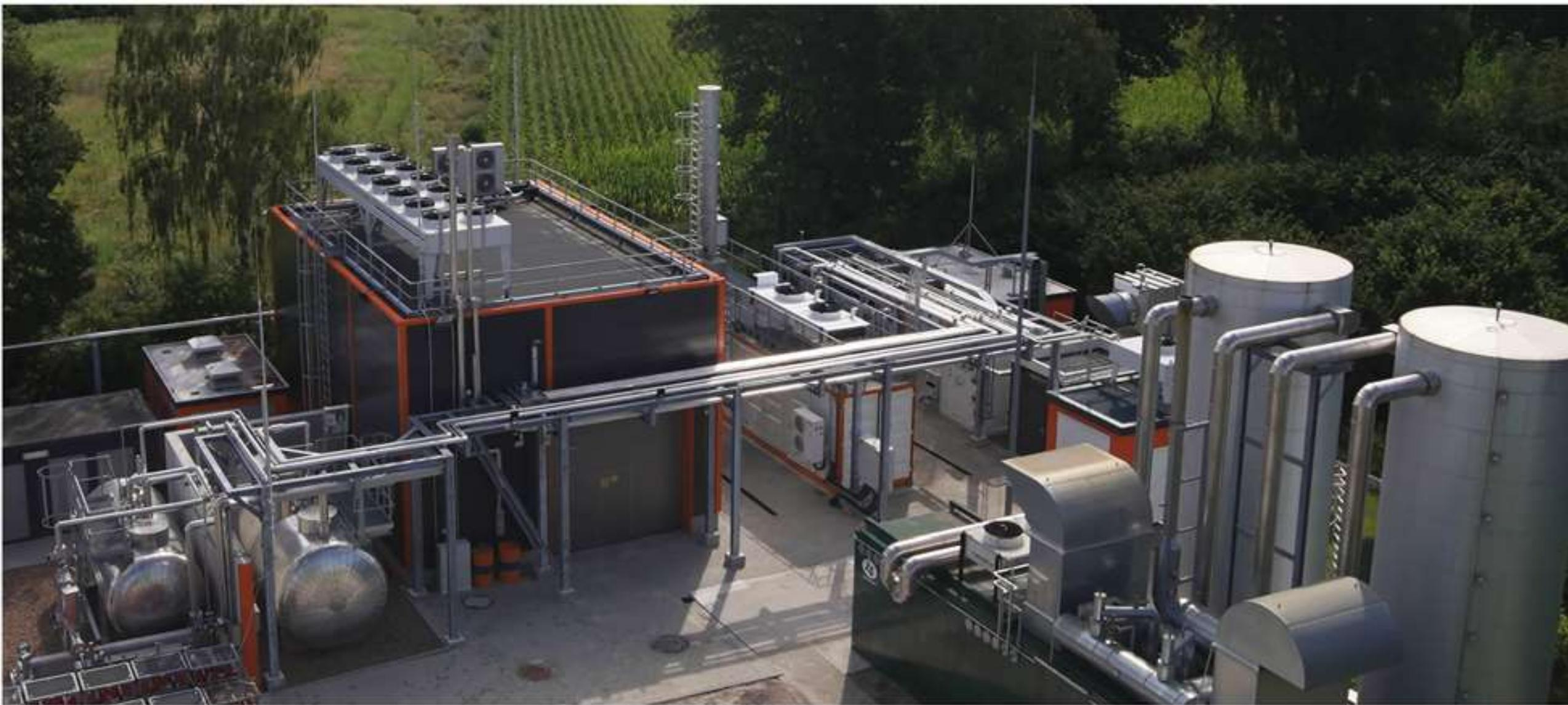
Fig. 24 Actual site of the 350 tpa of SAF production plant at Werlte in Germany, including the electrolysis system that forms the core of the plant
