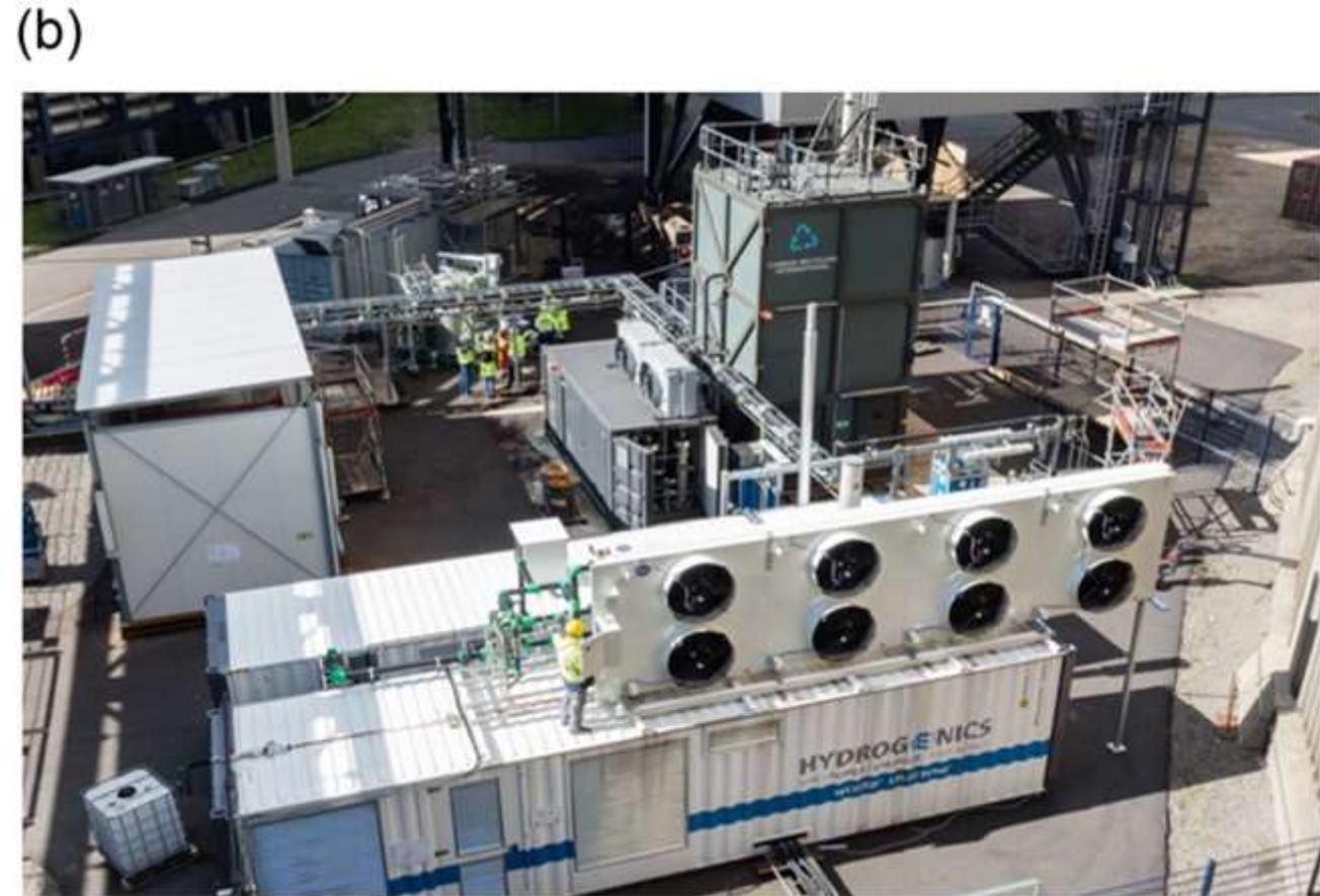
Fig. 19 (a) Schematic of the MefCO<sub>2</sub> plant and (b) the actual pilot-scale MefCO<sub>2</sub> plant (right) at RWE's lignite-fired coal power plant in Niederaussem, Germany.
